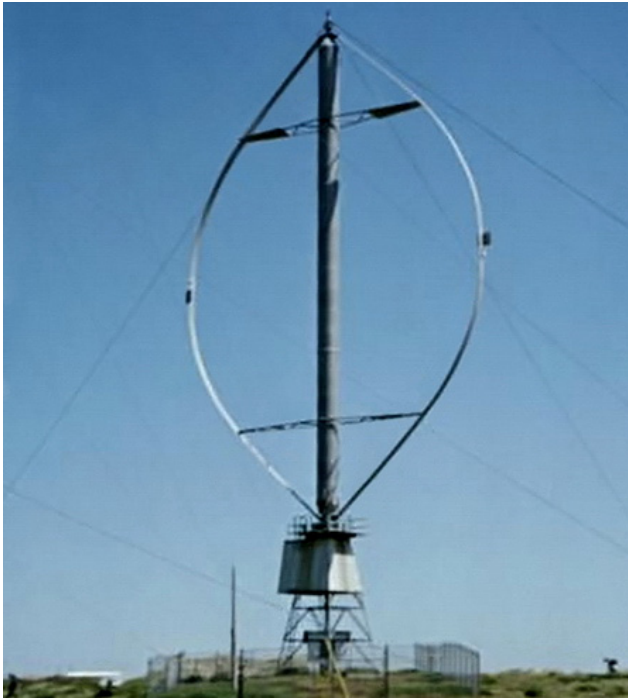
Figure 1.5. An example of a Darrieus wind turbine.
