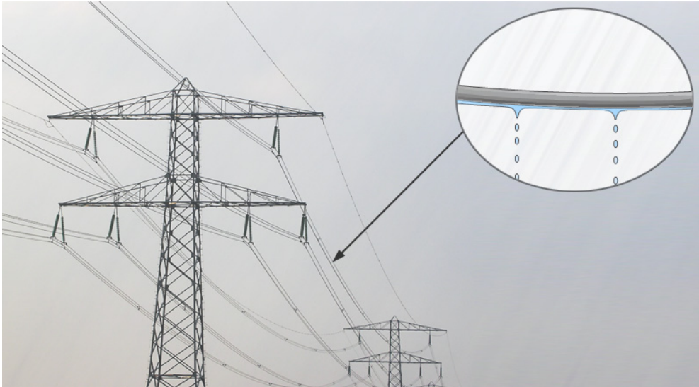
Figure 4.12. Taylor cones formed as on a high voltage overhead line.
