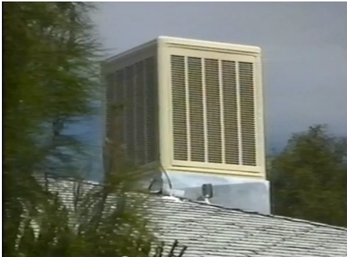
Figure 2. In areas of the United States where humidity tends to run high in the summertime, evaporative cooling is not the best way to stay cool; in the West, it's a very good choice.
