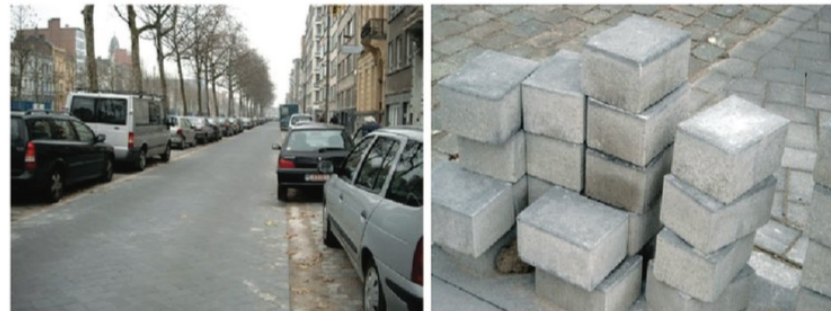
Figure 4. Separate parking lanes at the Leien of Antwerp with photocatalytic pavement blocks [15].
