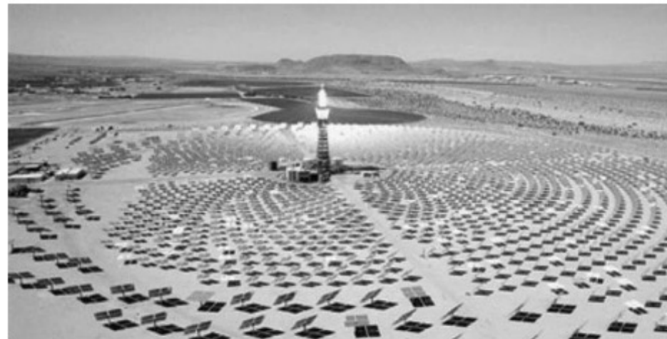
FIGURE 10.6 Photograph of the Solar Two central receiver plant (source: www.energylan.sandia.gov/sunlab/Snapshot/STFUTURE.HTM ).
