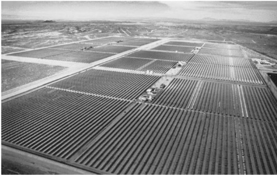
FIGURE 10.2 Photograph of a SEGS plant (source: www.energylan.sandia.gov/sunlab/Snapshot/TROUGHS.HTM ).
