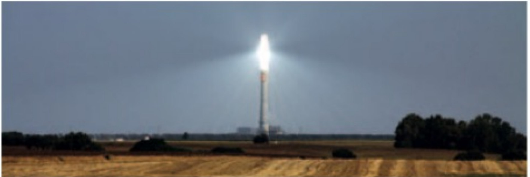
Photo 3.1 The Gemasolar power tower near Sevilla (Spain)
