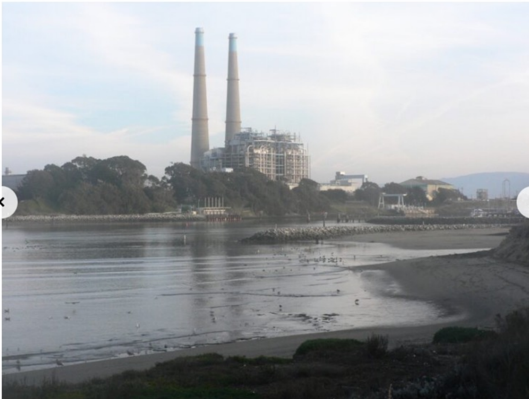
The Moss Landing battery energy storage project began operations in December 2020. Image courtesy of David Monniaux.
