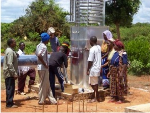
Figure 2. Local people helped install the solar icemakers.
