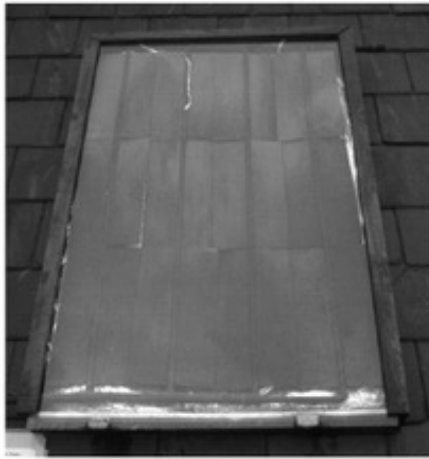
Figure 4-7 A home-made clip fin collector.
