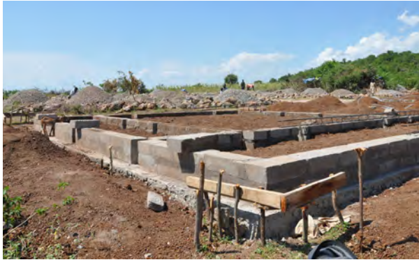
Images of foundation under construction.
