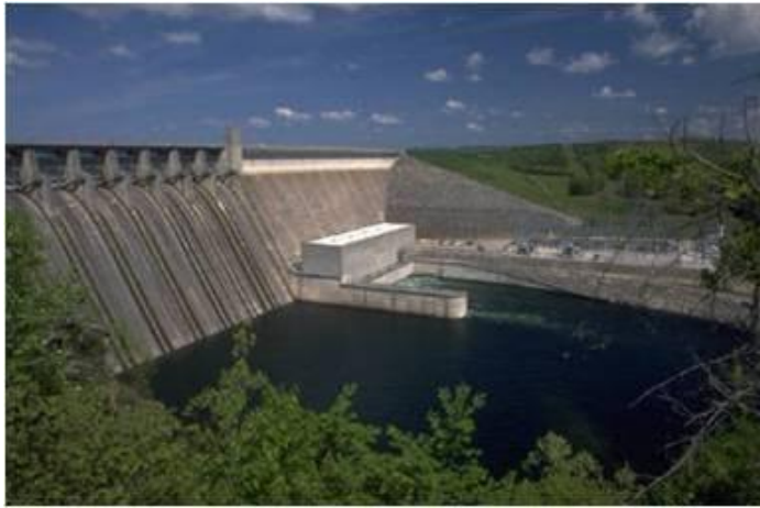
Courtesy of City of Tallahassee, Florida, Copyright 2001
