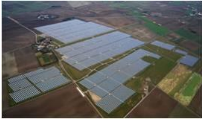
Source: Strasskirchen solarpark (54MW)
