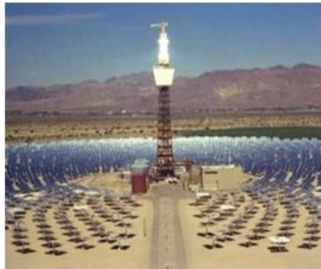
Parabolic mirrors focus the sun's rays onto the receivers
