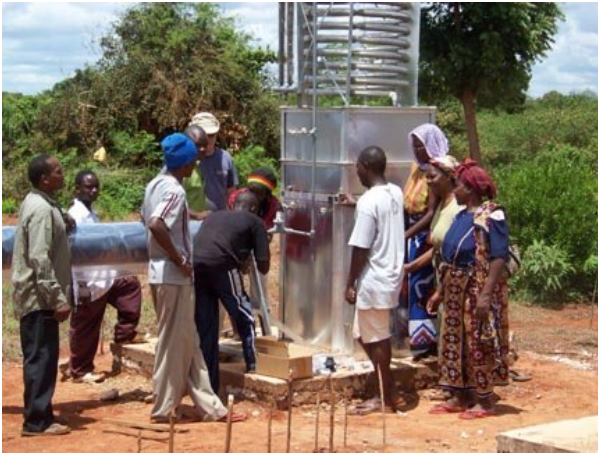
Figure 2. Local people helped install the solar icemakers.
