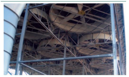
Photo 8.3 Dry cooling of the integrated solar combined cycle plant at Ain Beni Mathar, Morocco
