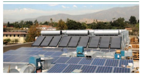
Photo 4.7 An installation of solar PV and thermal collectors on the same roof
