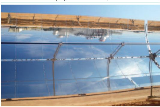
Photo 8.4 A parabolic trough and, reflected, the power block of the Integrated solar combined cycle plant at Ain Beni Mathar, Morocco
