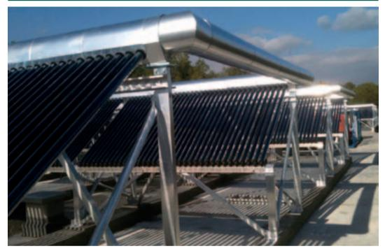
Photo 8.6 Experimental generation of electricity from non-concentrating evacuated tubes
