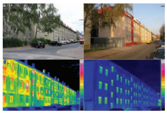
Notes: Top photos show the building before and after the refurbishment. Bottom images show infrared visualisation of the heat losses before and after the refurbishment.
