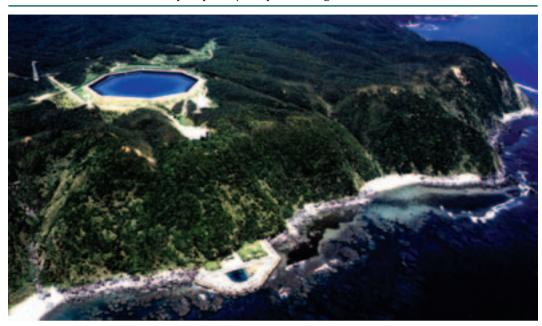
Photo 11.1 Okinawa's pumped-hydro plant using the ocean as lower reservoir
