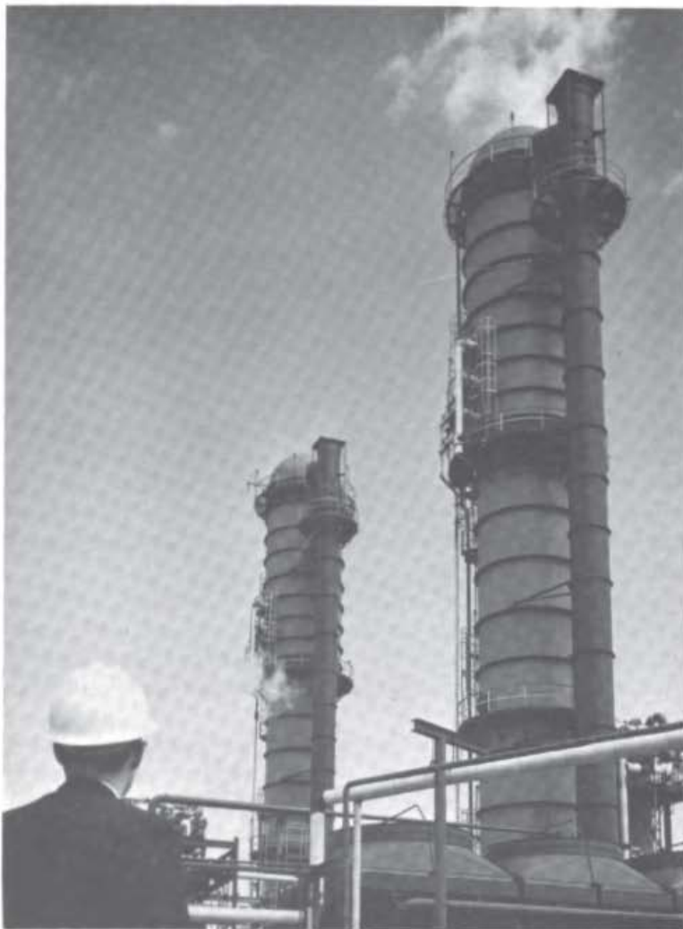
Figure 12-32 Two duplicate single-column distillation units for the separation of ethylbenzene and styrene each using 70 Linde sieve trays. ( Dow Chemical USA, Midland, Michigan. )
