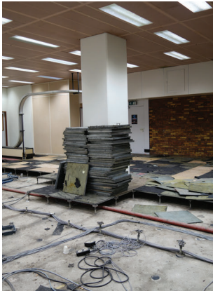
FIG 2.73 Removing a raised office floor for reuse
