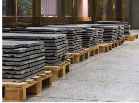
FIG 2.72 Carefully removing ceramic floor tiles for reuse
