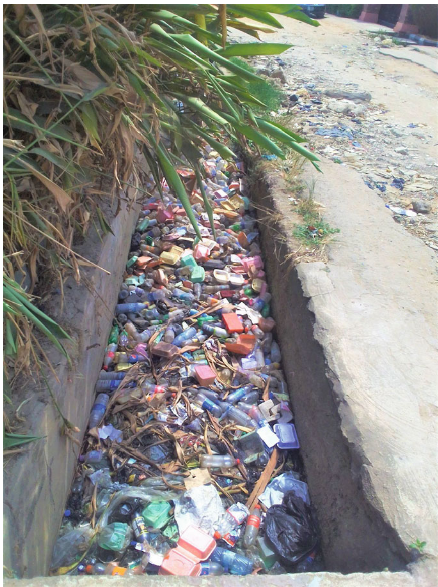
Fig. 10.8 Plastic waste blocking drainage on a street at Okota, Lagos, Nigeria. May 2022
