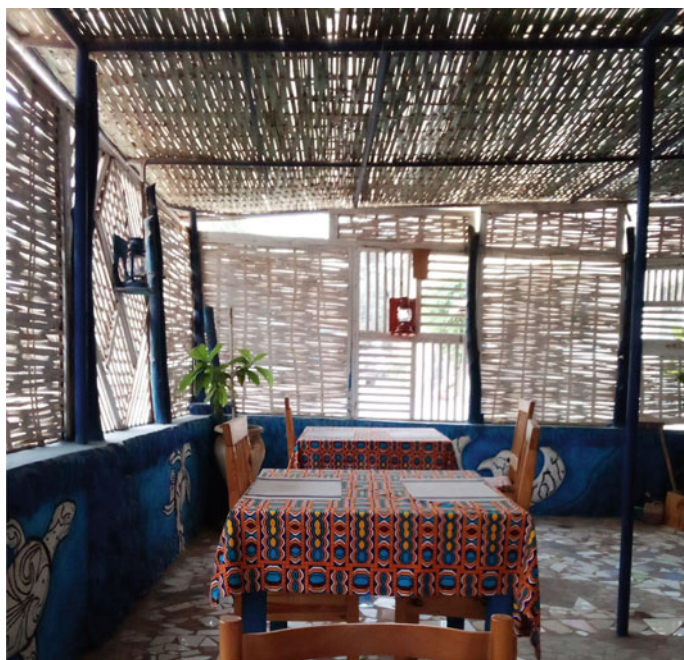
Fig. 3.9 Natural fiber used for ceilings and windows of a restaurant in Dakar, Senegal, December 2019
