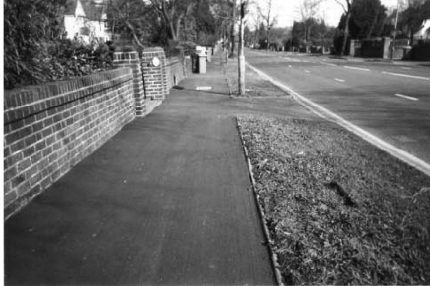
Figure 7.2: Pathways in Walsall in the UK have been resurfaced using a micro-asphalt product (Rejuvoflex) that contains waste tyre crumb. Reproduced with permission from the WRAP Quality Protocol, Waste and Resources Action Programme, Banbury, UK.
