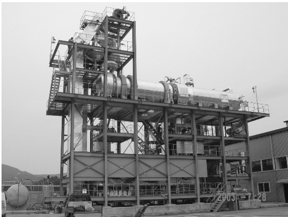
Figure 15.14 Photograph of the Reentech catalytic cracking process in Korea. The Reentech process converts mixed plastics (e.g. PE, PP, PS) into gasoline, kerosene and diesel fuel. (Courtesy of Reentech, Korea)
