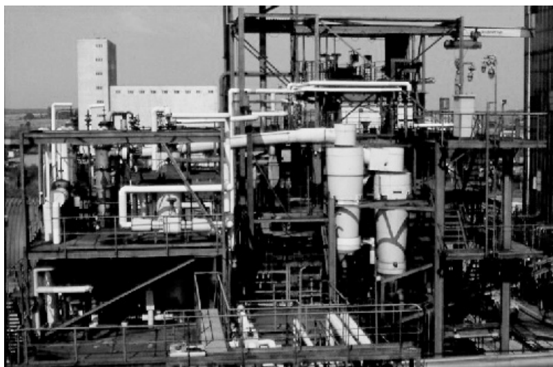
Figure 17.8 View of the Grimma plant for feedstock recycling of whole tires, in front two cyclones to separate the carbon black
