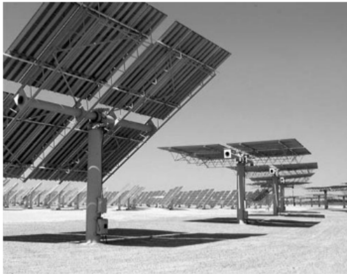
FIGURE 3.22 Detail of a heliostat.
