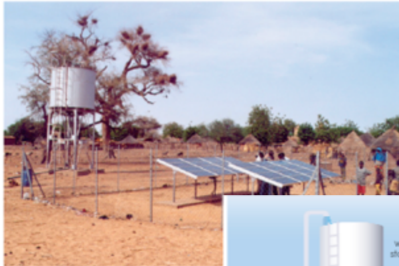
Figure 5.27 PV for a village water supply in Niger (
