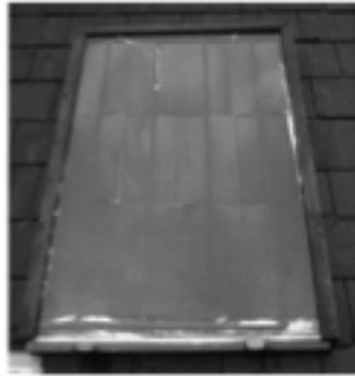
Figure 4-7 A home-made clip fin collector.
