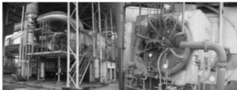
Fig. 2. View of the Barreiro power plant boiler (left photo) and detail view of the fuel feeding system in the boiler (right photo), with the central hole (open tube) used for wood tar injection, and the main round tube used for steel furnace gas injection.
