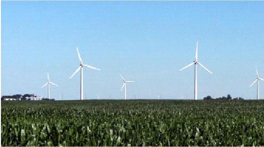
Figure A.4 A view of wind mills [2].
