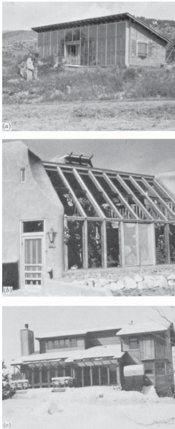
Figure 14.10.2 (a) The Odeillo single-family residence utilizing collector-storage walls. (b) Residence in Santa Fe, NM. (c) Residence in Golden, CO. (d) Monastery in Pecos, NM. (e) Waiting room of the Vielha Hospital, Catalonia, Spain. (f) Apartment buildings in Villefontaine, France.
