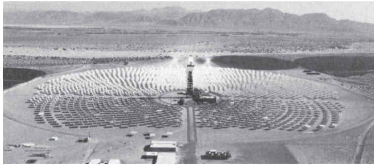
Figure 7.15.1 Solar One, a central receiver collector system. Photo courtesy of Sandia Laboratories.
