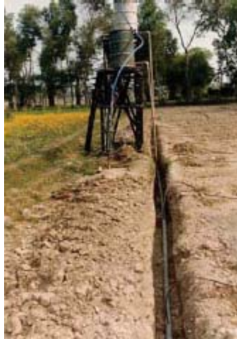
Fig. 7.6 Main and lateral laying
