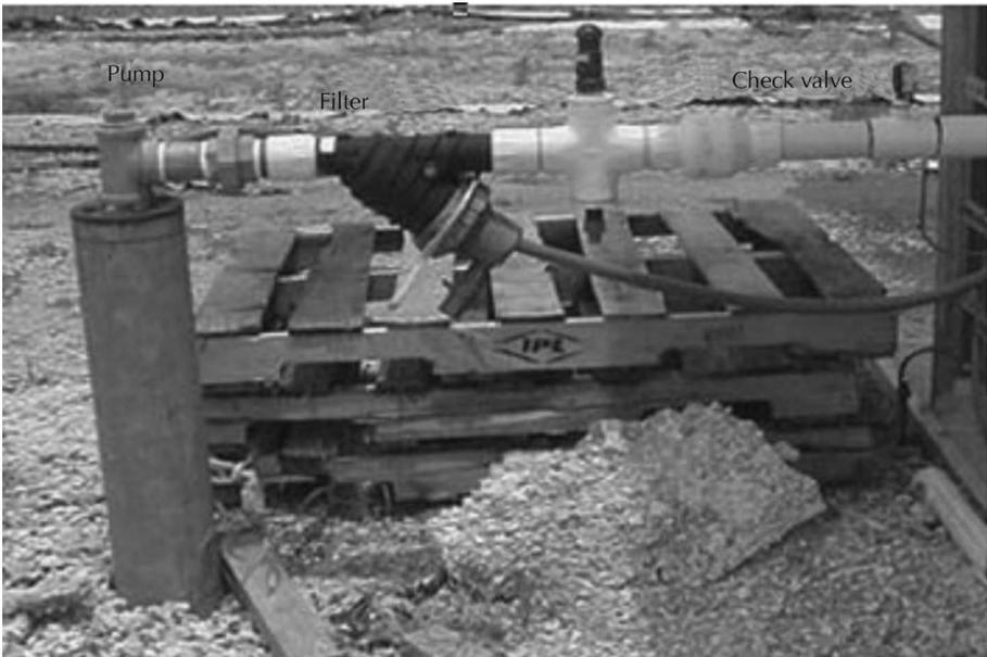
Water source, pump, and check valve assembly.
